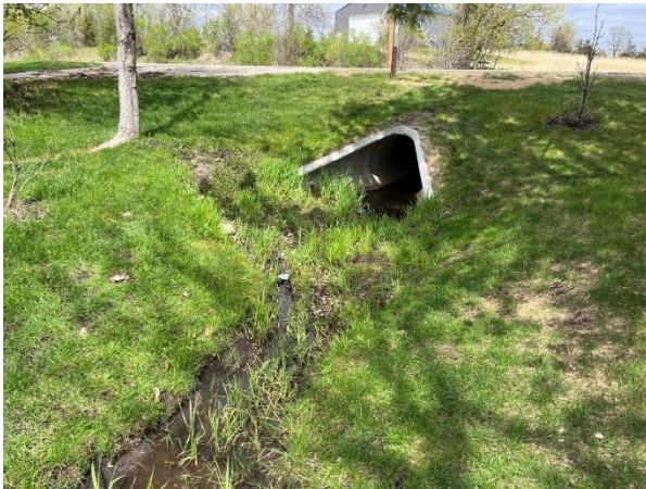
County Rd 47 Culvert Outlet - Before
