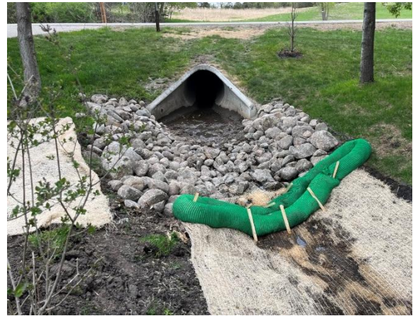
County Rd 47 Culvert Outlet - After
