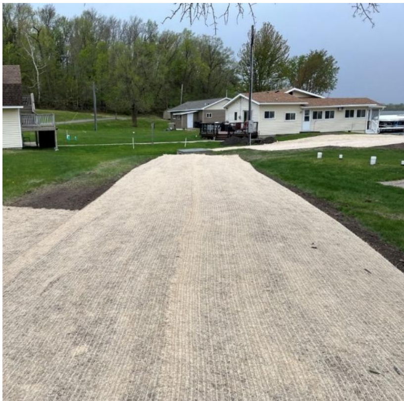
Constructed swale directing water to existing catch basin
